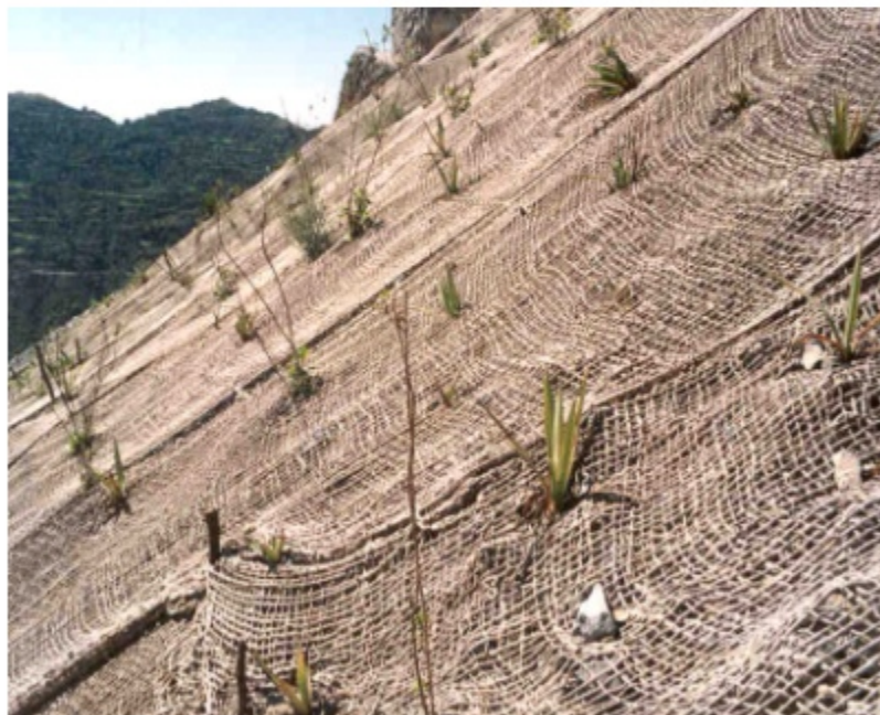
Fig. 8.1 View of geotextile used for topsoil stabilization and soil moisture conservation
