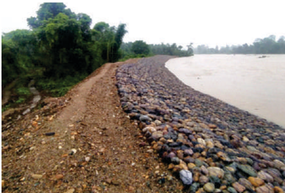
Bank revetment work Sile village, East Siang District, Arunachal Pradesh
