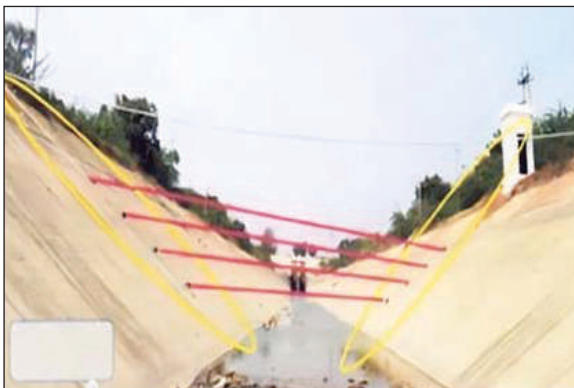
SCADA based canal control system using flow sensors with GSM supported communication over Narmada canal of the Sardar Sarovar Project
