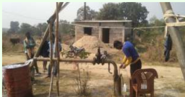
Ground Water Exploration activity under NAQUIM was conducted in Maliberuar village of Jharsuguda district, Odisha, having a discharge of 2.18 lps.
