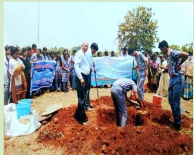
Pits to conserve rainwater.
