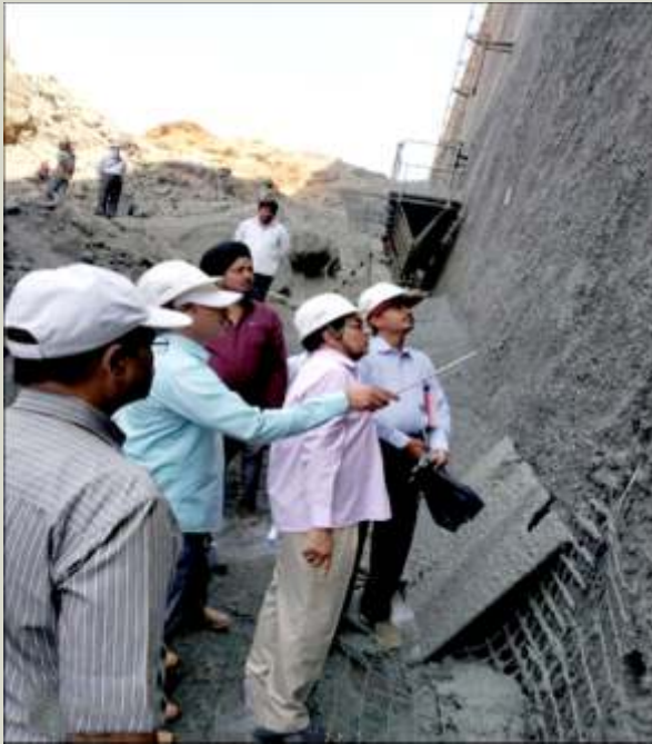
Inspection of Shotcreted Surface
