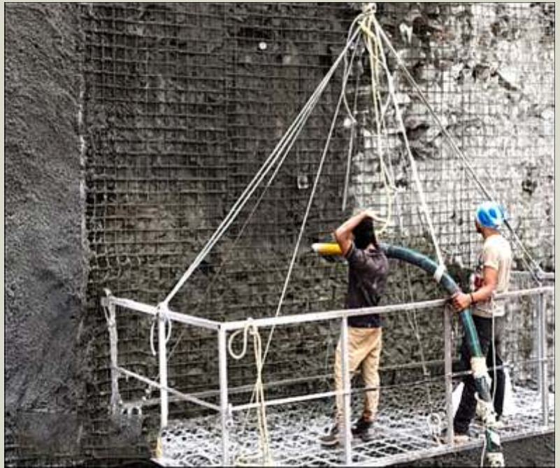
Shotcreting in process at Site
