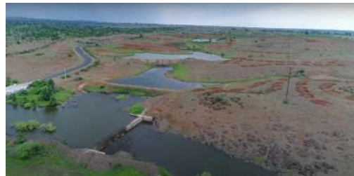
Pond work under Krishna Rejuvenation 2019-20
