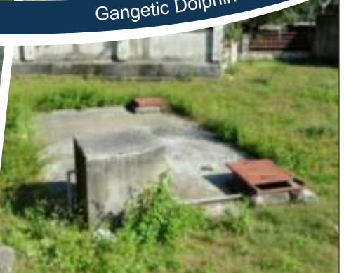
Rainwater Collection Tank at Vaishno Devi
