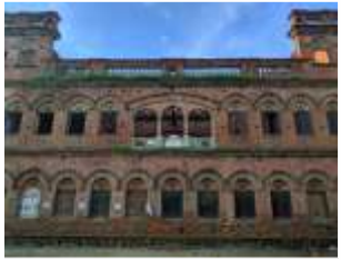
Abandoned Colonial Warehouse [Mirzapur]
