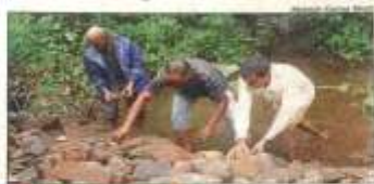
STREAM OF CONSCIOUSNESS: Villagers conserve a river check-dam using house builders to retain rainwater.
