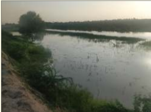
Renovated Tank Pochannapet GP of Bachannapet Block.
