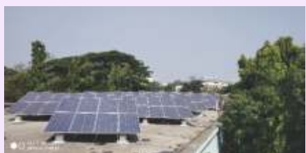
DOHI Building Roof Top
