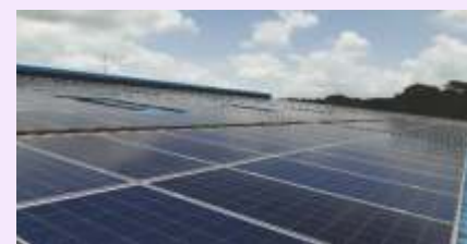
Multipurpose Wave Basin Hanger Roof Top
