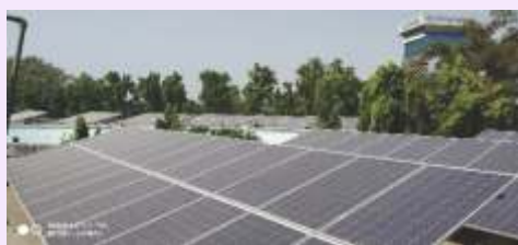
DOHI Building Roof Top
