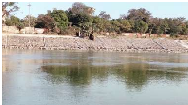
Fig: Feeder Canal Inspection
